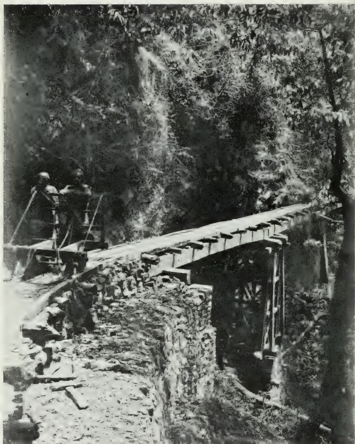
FIG. 159. WOODEN TRAMWAY AND BRIDGE : INDIA.
